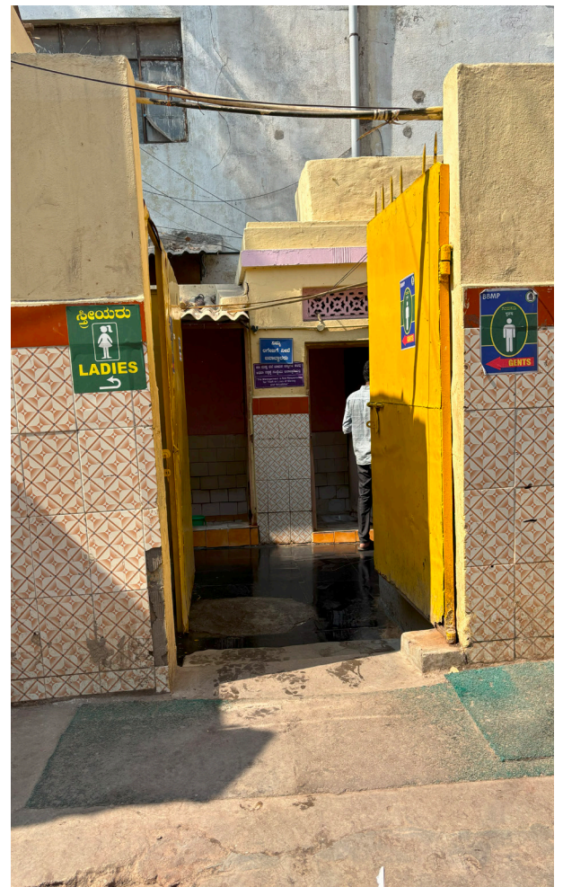
A public toilet in Chickpete, with universal symbols in green color affixed on the walls outside.
